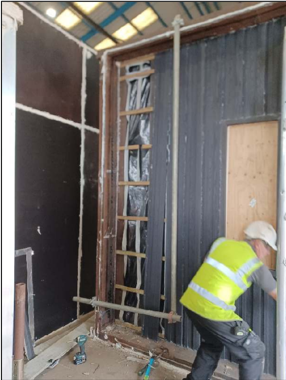
PLANKS REMOVED FROM SUPPORT FRAME
