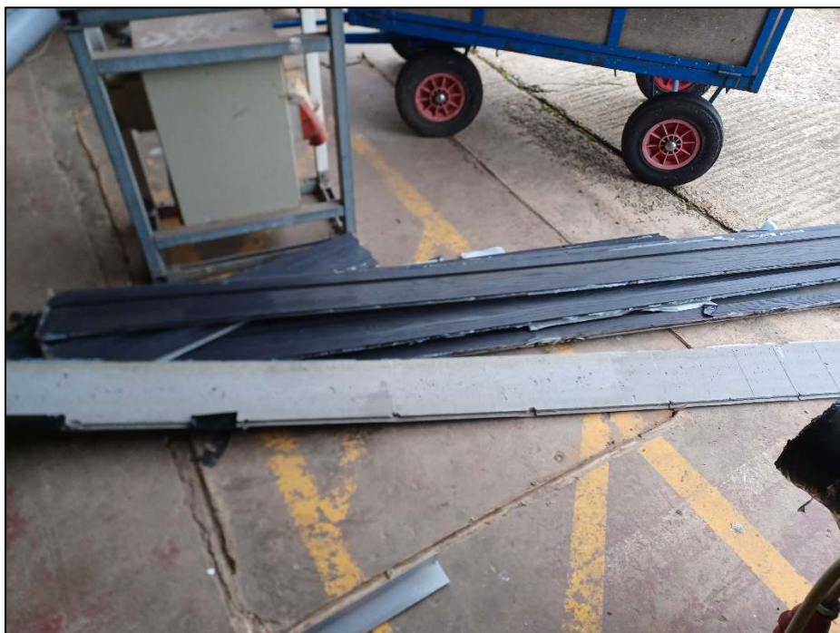
PLANKS REMOVED FROM SUPPORT FRAME
