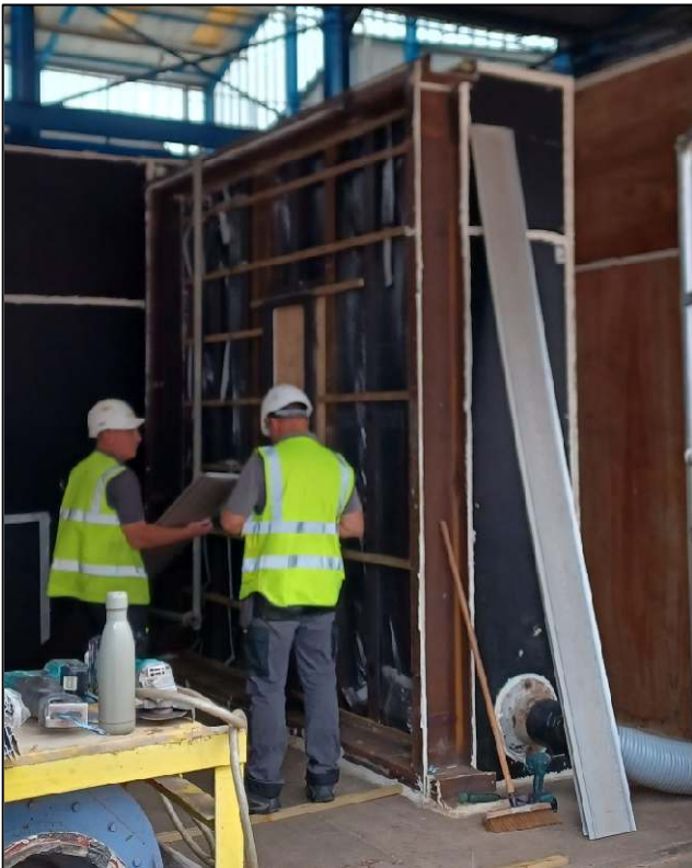
PLANKS REMOVED FROM SUPPORT FRAME
